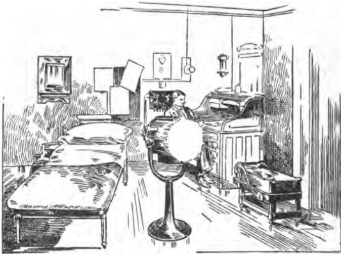
One of the Rooms for Electrical Treatment—Invalids' Hotel.
